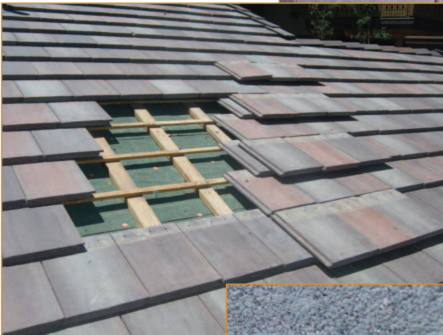
Photo 11 – The vertical battens must be nailed in order to transfer the wind load; after that, the horizontals must be nailed to the verticals, then the tiles to the horizontals. If not, there must be sufficient weight to resist wind uplift. Roof edges will have sufficiently increased uplift loads and will require additional fastening or clipping.
