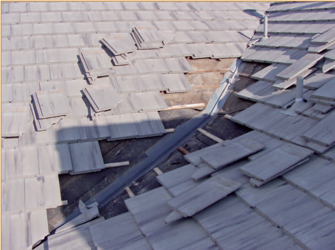
Photo 7 – This valley is constructed with horizontal battens that will trap debris. The use of a closed valley requires that tiles be removed in order to perform the required maintenance.
