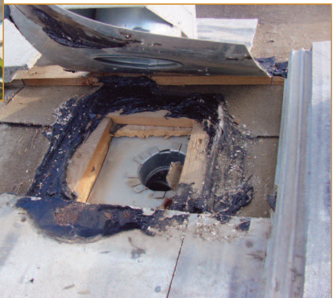
Photo 6 – The lapping of flashings and all moisture-management materials should ensure that water is directed down, out, and away from the roofing felts. In no case should mastic or sealant be relied upon to correct deficient construction.
