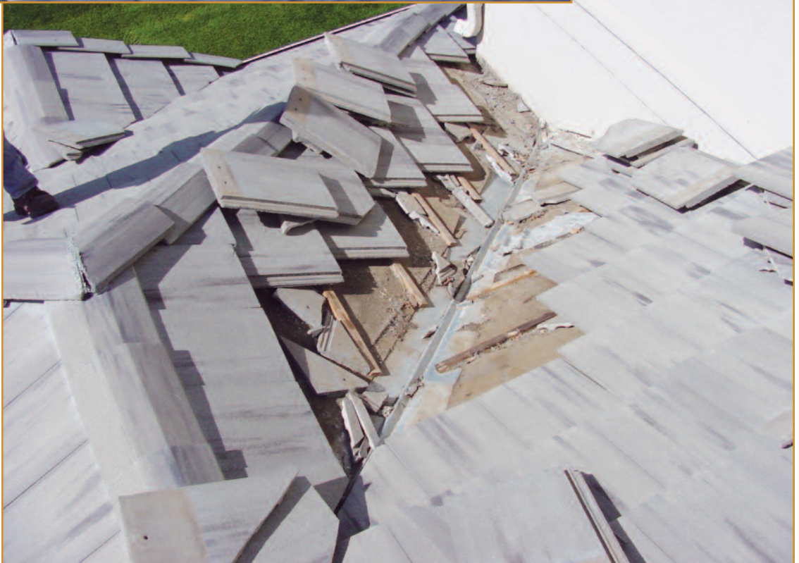
Photo 8 – Poor valley design by the architect is shown here. The design directs water into the vertical unit-demising wall and allows buildup of ice and snow against the cladding.
