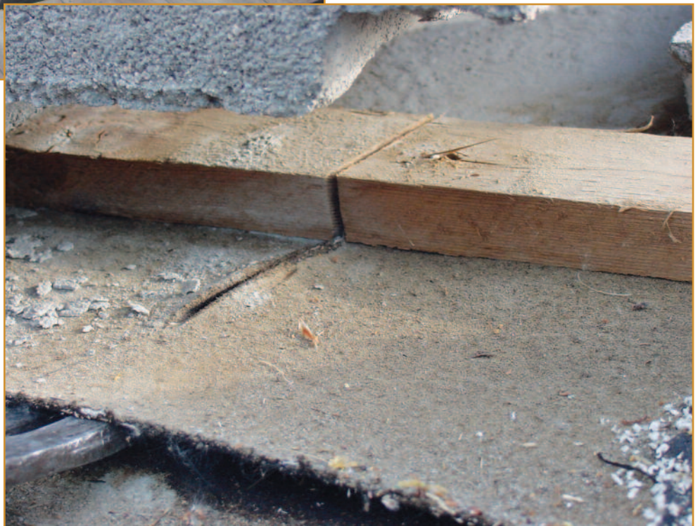
Photo 12 – Horizontal battens require that water drain to the slots. In order for that to happen, water must back up and work its way to the drainage slot. In the photo below, the slot appears to have been cut after the installation of the batts; this creates an opening in the roofing felts for the water to drain through. Vertical battens with the horizontal battens applied over the top are preferred over this type of installation because they create a direct and uninterrupted path to the edge of the roof.
