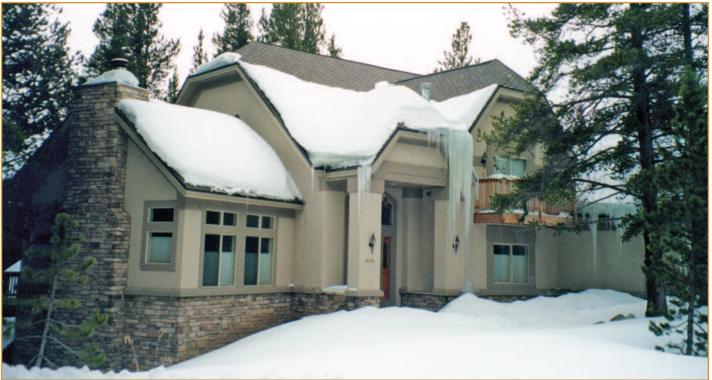
Photo 2 – Roof layout and an understanding of ice and snow accumulation are extremely important and should be fully considered by the design and construction team prior to applying the roofing and integrating the building veneers.
